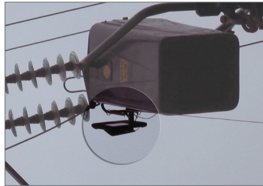
Power Line NDT
